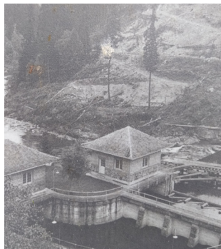
Photo Credit: Tacoma Power
