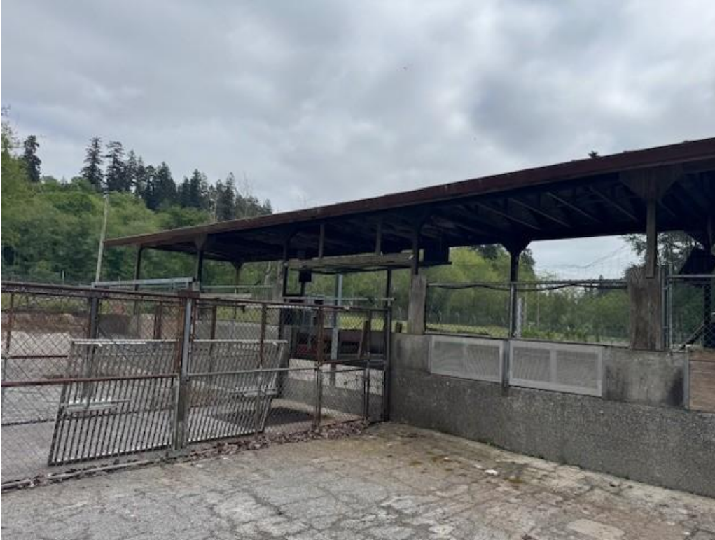
09 – Head of Pond 15 (showing raceway fencing and fencing over concrete wall)
